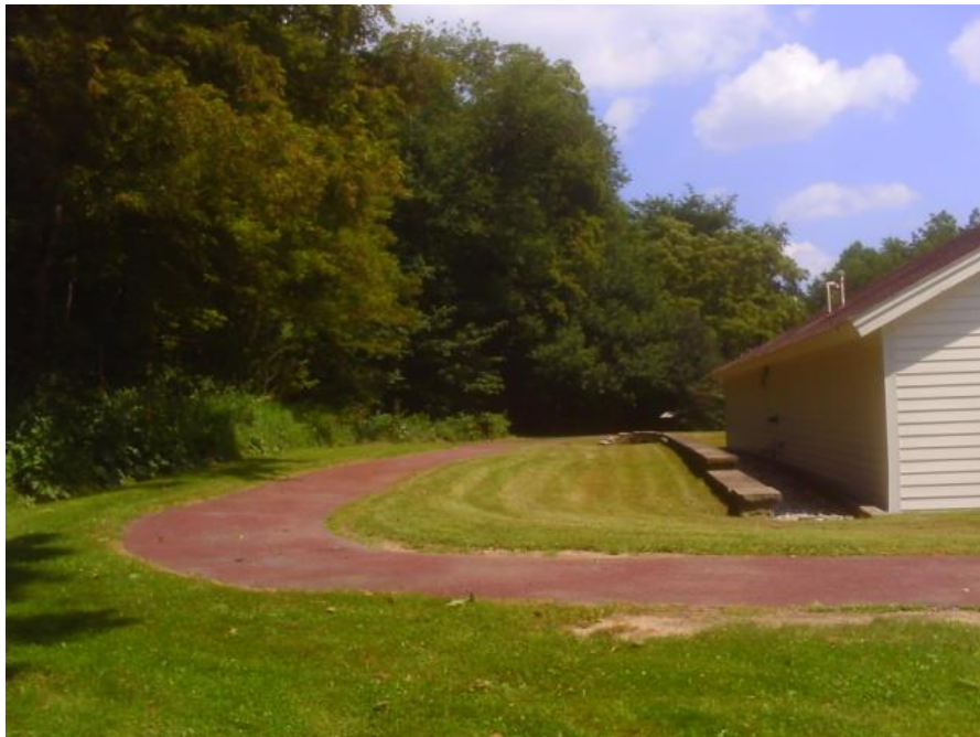
Figure 20: West Side of Engine House # 6.
