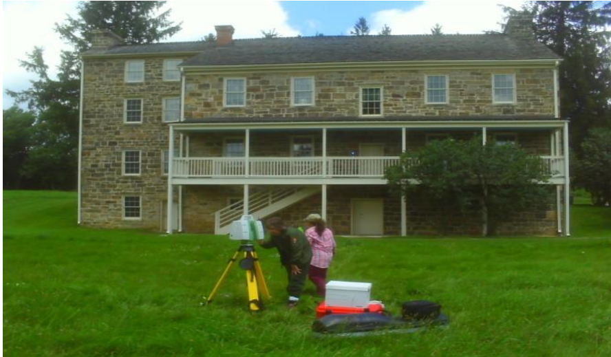
Figure 23: Back View of Lemon House at Station 01
