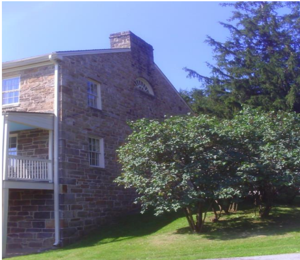
Figure 26: View of Lemon House for Station 04.
