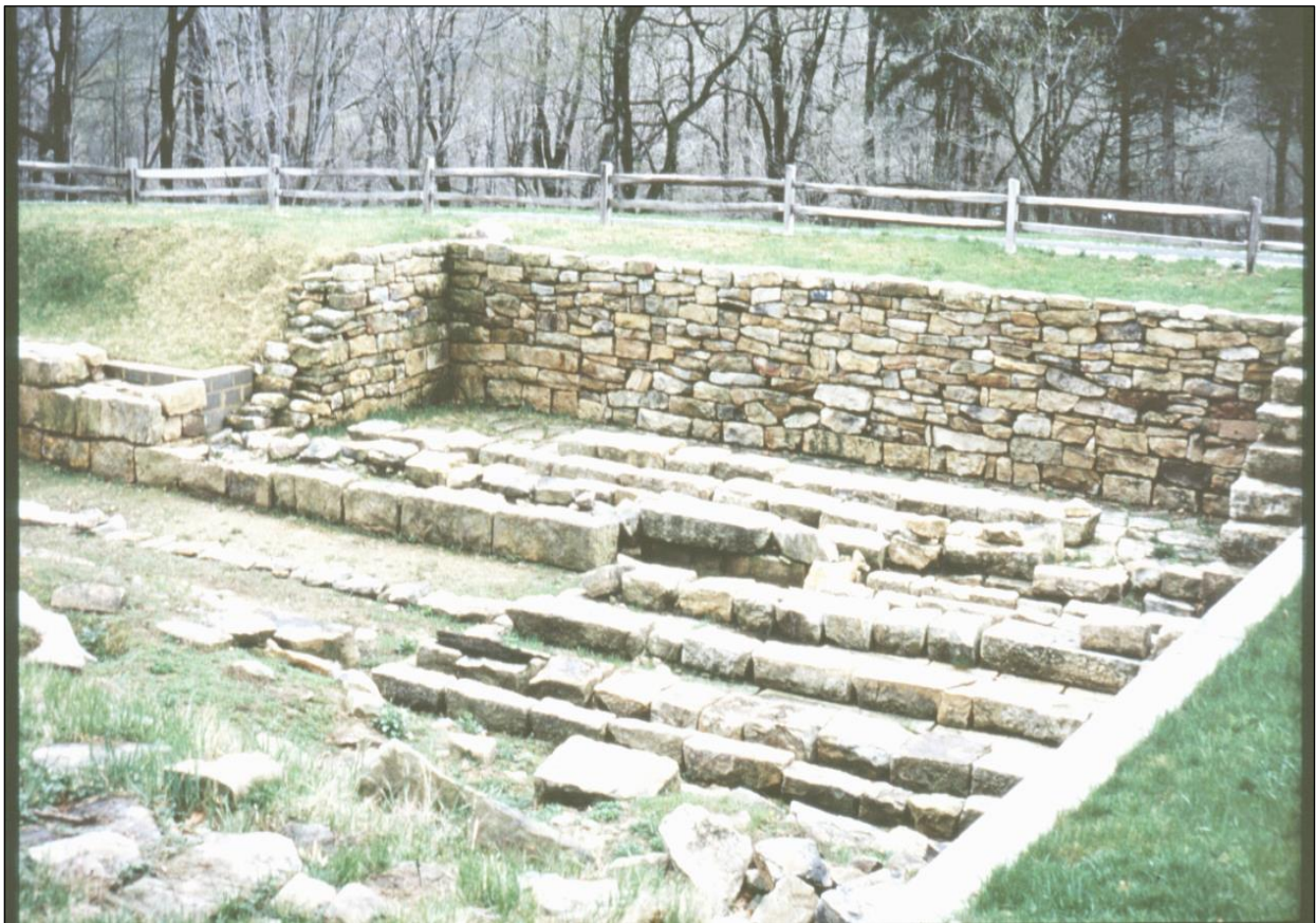
Figure 10: Remains of Engine House 6 Foundation Stones (Courtesy of NPS)
