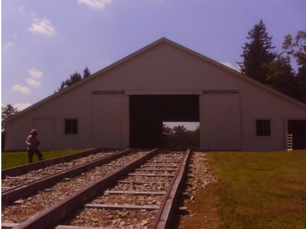
Figure 21: Back View of Engine House #6
