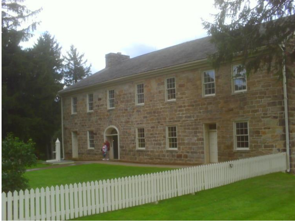
Figure 25: Front View of Lemon House for Station 03.
