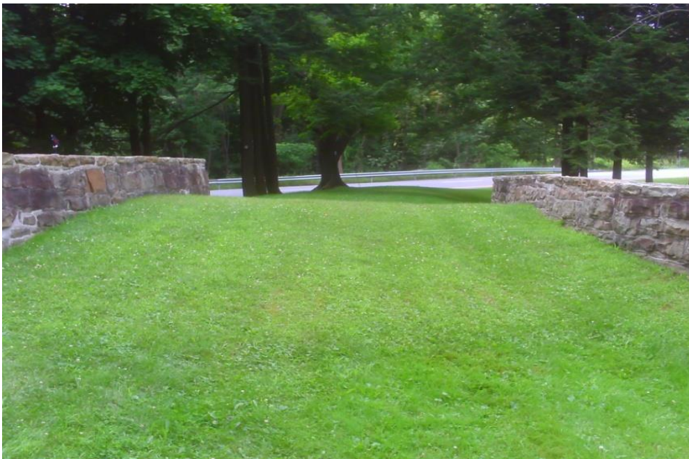
Figure 18: Station 04 Bridge Path view
