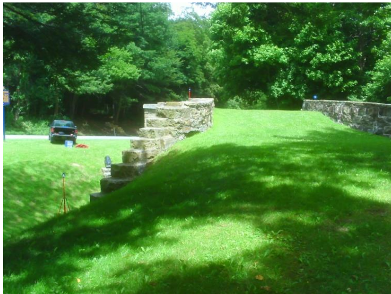
Figure 16: Station 02 Target Positions for Skew Arch Bridge.
