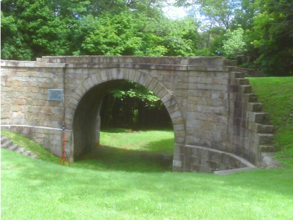
Figure 17: Station 03 Targets at Skew Arch Bridge.
