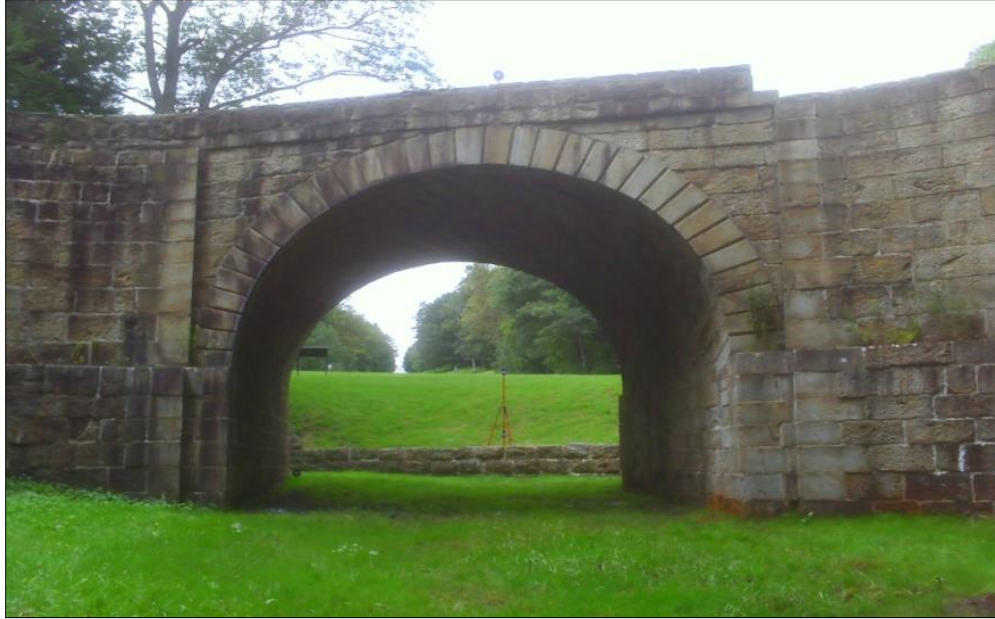
Figure 14: Image showing center target locations for Station 01 Skew Arch Bridge.
