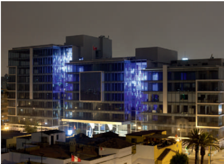
Aronas chandeliers by Cinimod Studio were used in an office in Lima, Peru.
