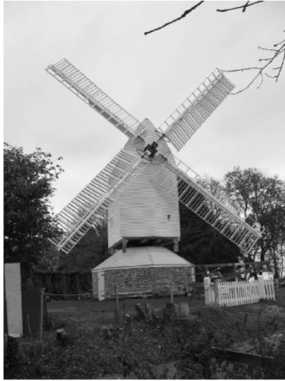
Figure 1.10 Post mill ( http://en.wikipedia.org/wiki/File:Oldland_Mill.jpg )
