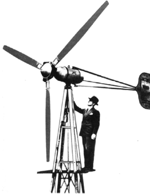
Figure 1.14 Jacobs turbine (Jacobs, 1961)
