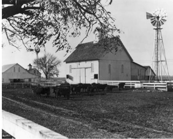
Figure 1.13 American water-pumping windmill design (US Department of Agriculture)
