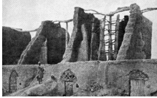
Figure 1.9 Seistan windmill (Vowles, 1932)
